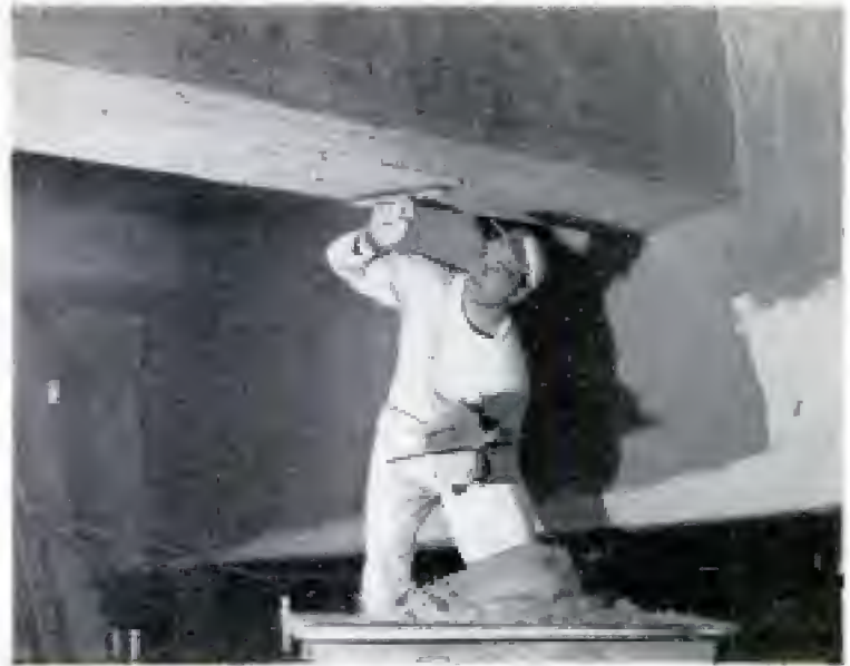
Plaster made with perlite instead of sand weighs only a third as much as ordinary plaster, is both decorative and fireproof
